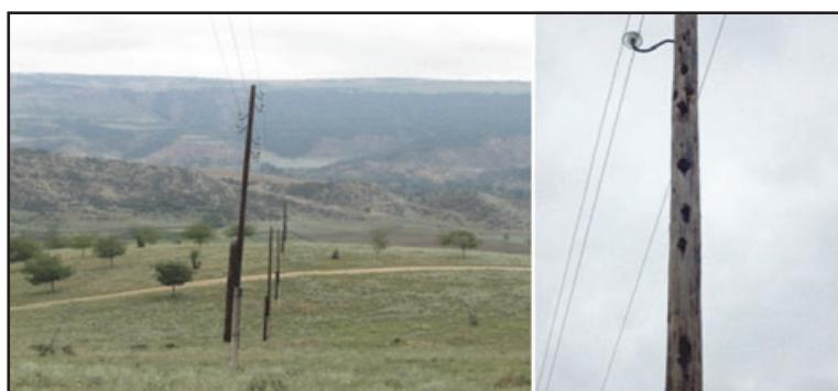
damaged poles were replaced by new ones, also wooden but well-processed and resin-impregnated. After that, cases of bird deaths in this section were not discovered.
