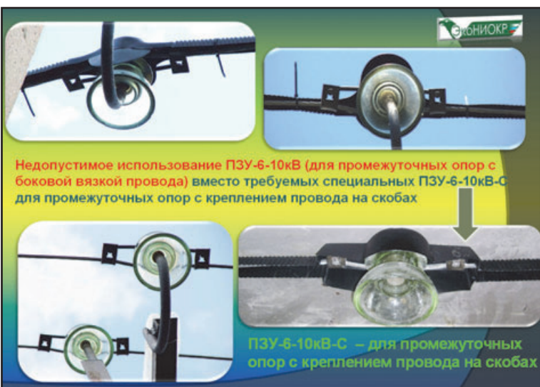
Fig. 10. Applying BPD-6-10 kV instead BPD-6-10kV-D.
